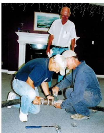
Photo – Repairing the floor Vern Willis & Dale Procnier
