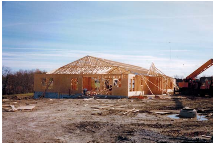
1998 - Construction of The Centre
